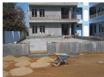
Foundation for Sports Ground
