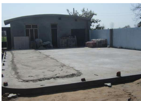
Foundation for Play Ground
